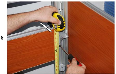
Adjust the brackets to the mark level (dot) showing on each post.
