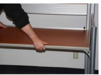
The 4 brackets are now locked at the same height and ready to receive the work top.
