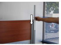
Insert each filler designed to hide the empty space on both posts B, as per pictures, right and left.
