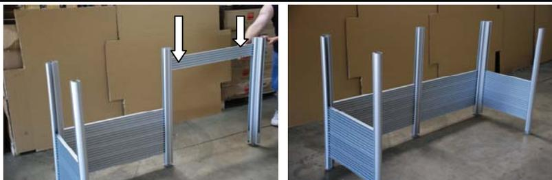
Slide (4) rail-panels 2 (36" W) in between linear post C and 2-way post B. Same with (4) rail-panels 1 (24" W) in between 2-way post B and last end-post A.
