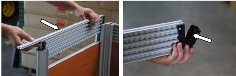
**TIP 1:** Identify panels that come with a pre-installed alu cap. They go on the top.
